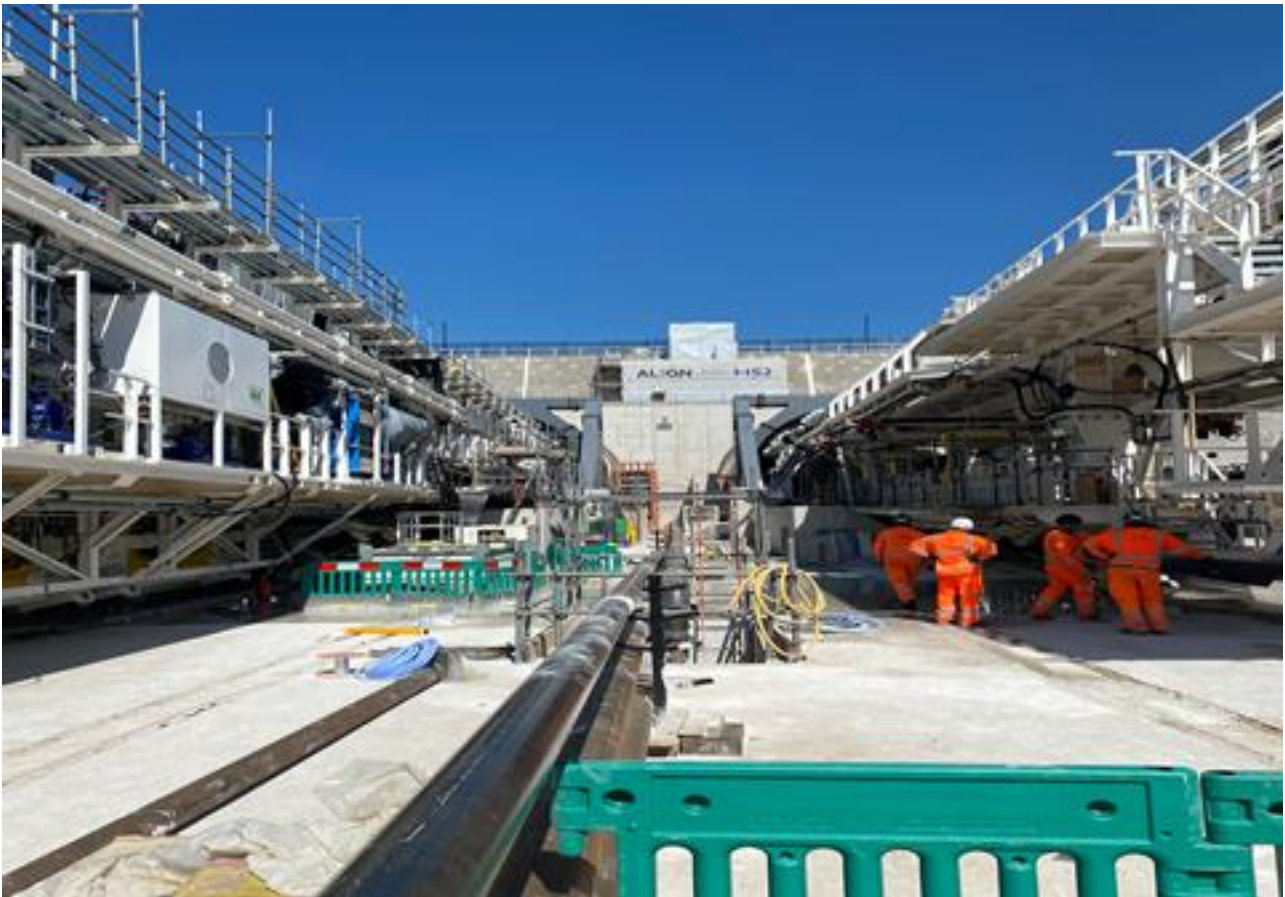
The first tunnelling machine at HS2's South Portal site just outside north west London was launched last month.
